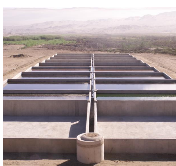
b) Typical drying bed array
