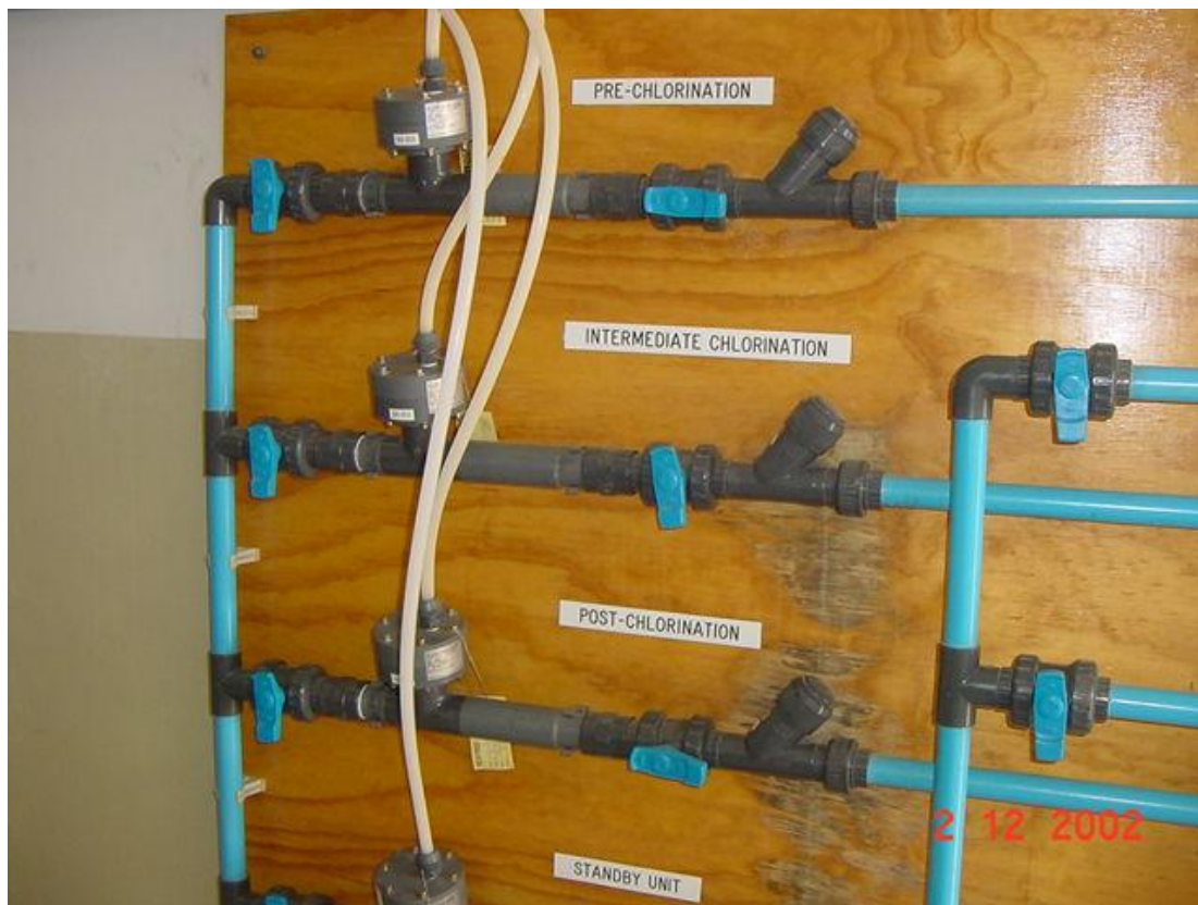
Figure 20: Typical gas chlorination board with multiple injectors
